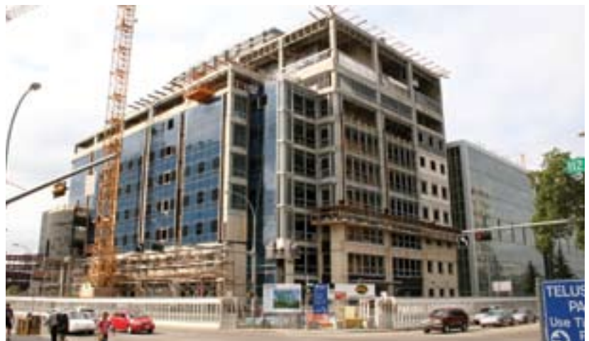
HRIF-East under construction, corner of 83 Avenue and 112 Street.
